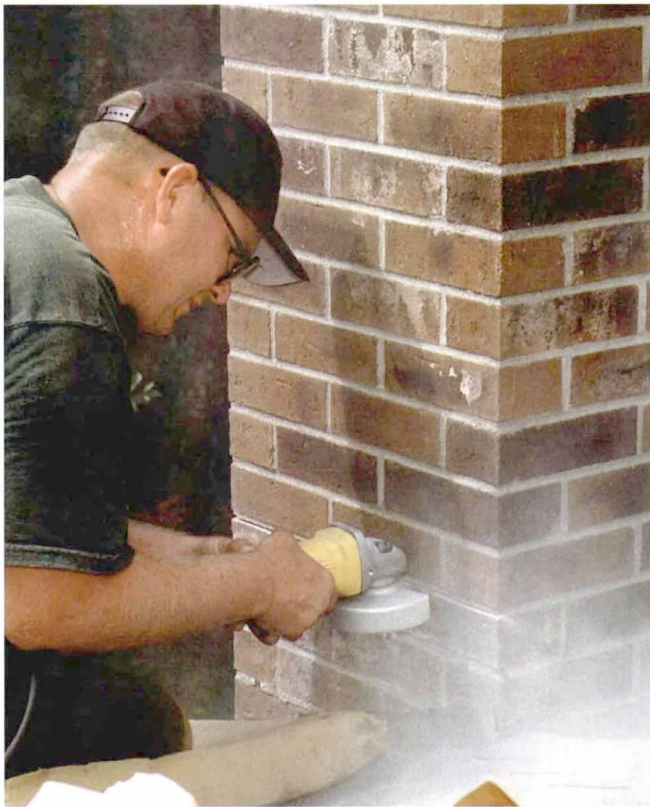
New counterflashing. When reflashing a chimney, the author grinds out the mortar for new counterflashing one course above the old. And yes, he should have used a mask or respirator for this work to protect his lungs.
