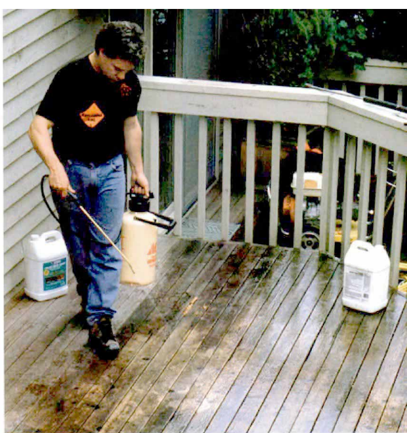
Cutting quickly through the crud. Applied using a garden sprayer, a specially formulated deck cleaner dissolves dirt and oxidation and kills mold and mildew on contact.
