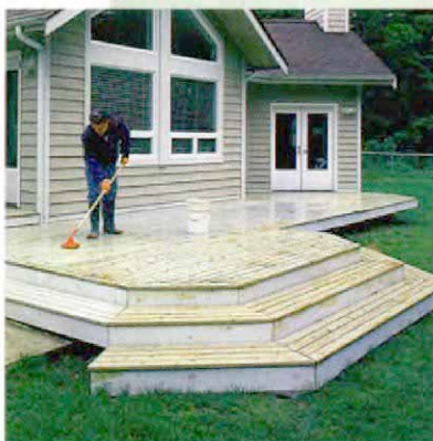
Stripper is applied with bucket and brush.
