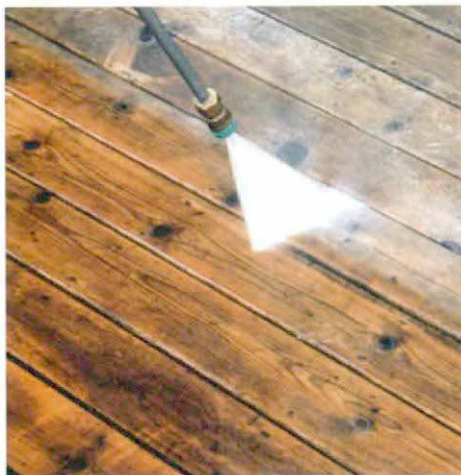
Be careful with the pressure washer. For maximum cleaning with minimal abrasion, the author holds the 15° spray tip 6 in. to 9 in. above the deck and gradually sweeps across the boards in a flattened pendulum motion.
