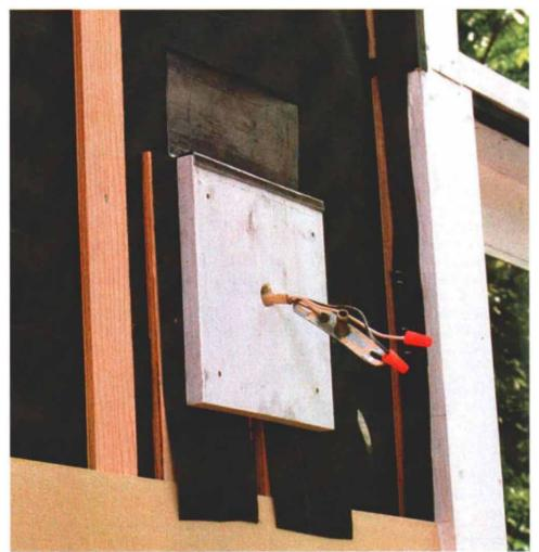
**If siding leaks at joints, let it drain.** The tar-paper splines under this light-mounting block both cover the furring strips and extend over the next lower clapboard to drain water away from the house.
