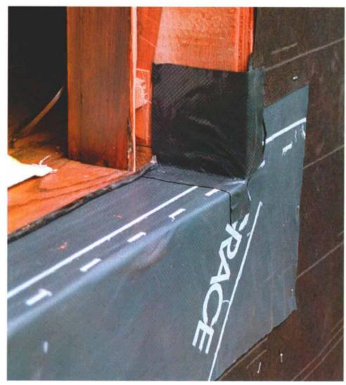
**First, flash vulnerable spots such as rough sills to drain water.** Note how the tar paper to the right of the opening laps over the top of the Ice & Water Shield flashing. In turn, the Ice & Water Shield laps the tar paper below.
