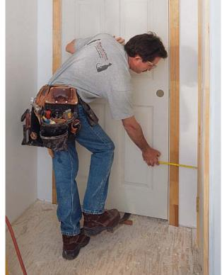
There's more to setting a door than plumb and level. Although setting a door plumb is ideal, it must also look parallel to adjacent walls or trim. A quick check with a tape confirms parallel.
