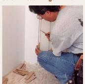
long screw that reaches through the jamb and into the trimmer. Often I replace two screws in the top hinge. I tighten the screws carefully because too much torque will cause a belly in the jamb and ruin the fit of the door. If I don't have the right-size screw, I remove the hinge from the jamb and countersink a screw behind the hinge, then reattach the hinge to the jamb.
