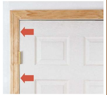
Even lightweight hollow-core doors can cause hinge deflection. Notice that the gap between door and jamb is larger above and below the hinge. Raising the door with a pry bar and nailing the casing to the wall behind the hinge corrects this problem.
