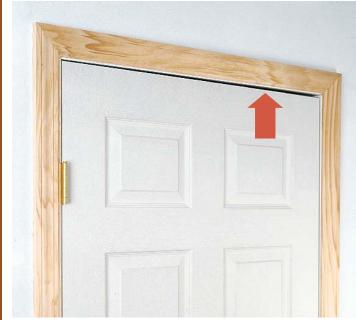
Wide head gap requires correction. Raising the hinge jamb or moving its bottom toward the opening's center will close this gap. Another alternative is to lower the jamb by trimming the bottom of the strike jamb.
