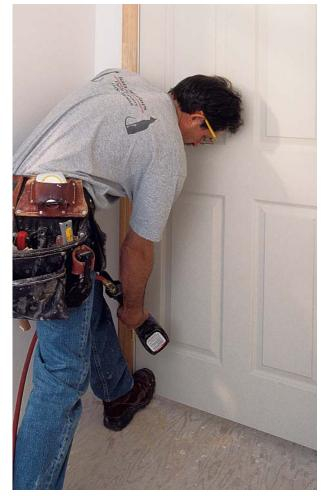
Correcting cross-legged jambs with a boot and tap. The fix when the door doesn't hit the top of the strike-side stop is pushing in on the bottom of the hinge jamb. If the door doesn't hit the bottom of the stop, simply moving the strike-jamb bottom toward the door is the cure.
