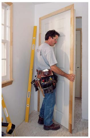
Casing the prehung unit is the first step. With no drywall irregularities to contend with, perfect casing miters are a snap. The author glues and nails the miters to ensure that they stay perfect.
