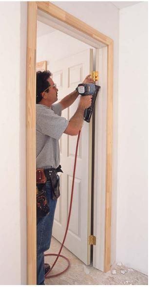
Tight miters are the only challenge on the stop side. With the door adjusted to the jambs, trimming the stop side is a matter of shooting in nails every 12 in.
