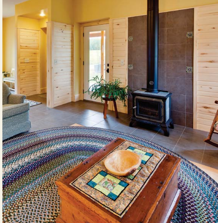
A woodstove in a tight house? Wagner has put woodstoves in many ultratight houses with no drafting problems. When using their clothes dryer, though, the homeowners have to crack open a window.
