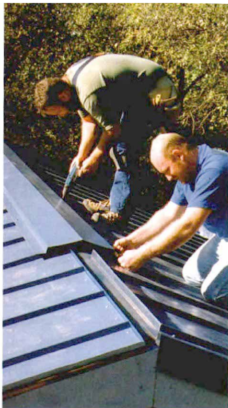
Chalklines guide ridge-vent installation. Marks are made on the roofing from a scrap of ridge vent, and lines are snapped between the marks (photo left). The vent is held to the chalkline and screwed down to keep it running in a straight line (photo right).
