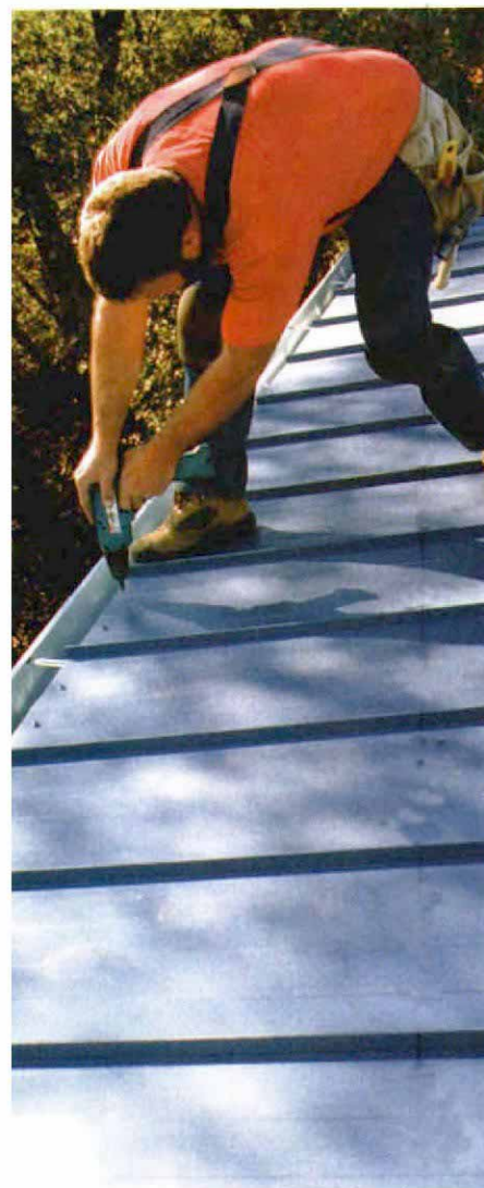
Screws keep the bottom edge flat. Gasketed screws are driven between the ribs of each panel along the bottom edge to keep the panel flat.
