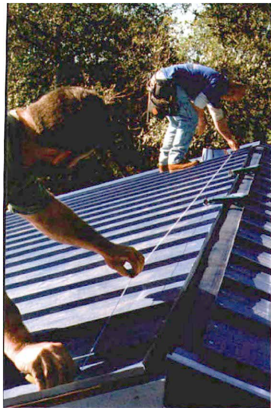
Chalklines guide ridge-vent installation. Marks are made on the roofing from a scrap of ridge vent, and lines are snapped between the marks (photo left). The vent is held to the chalkline and screwed down to keep it running in a straight line (photo right).
