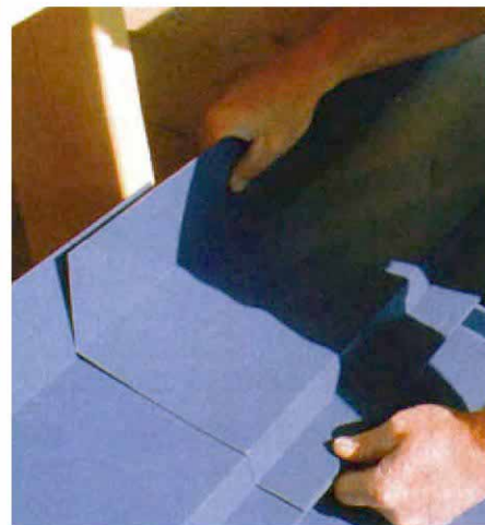
Overlap trim pieces in long runs. When a run of trim requires two or more pieces of trim, the pieces of metal are overlapped about 6 in. and then held in place with gasketed screws.
