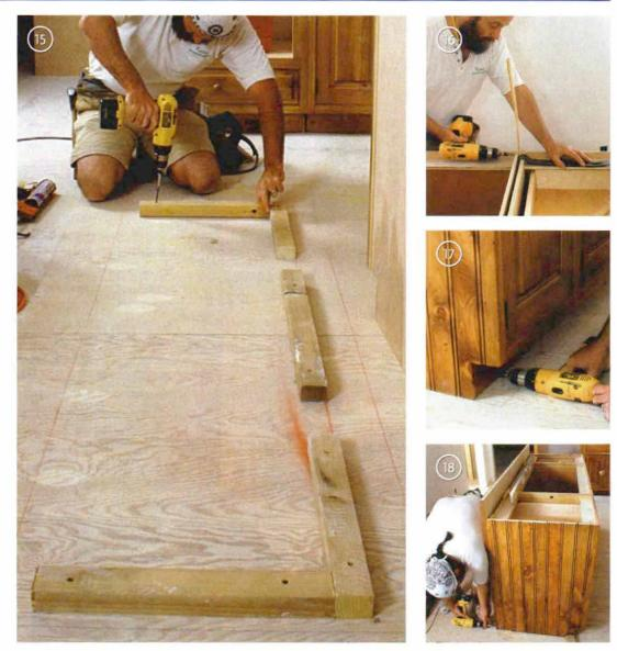
so checked the distance to the other cabinets. The corner cabinet was left loose with the idea that I could slide it up and out of the way when the countertop was installed and then drop it down for a precise fit on the granite counter.
