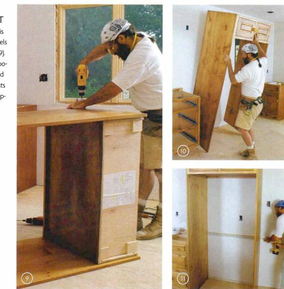
bled, I lifted it and rotated it into place (photo 10, facing page). Like most refrigerator cabinets, this one was deeper than the base cabinets. I plumbed and leveled the cabinet and then screwed the left side into the face frame of the adjoining base cabinet.
