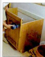
appliances. On the right side of the dishwasher, I installed a wine-rack end panel screwed to a 2x cleat on the wall.
