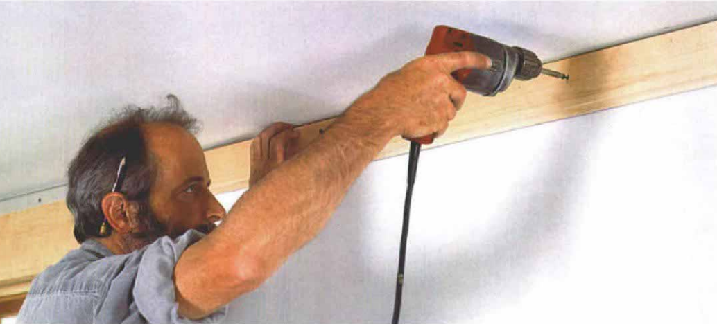
Backing trim makes a solid nailing surface for molding. Screwed into the framing, a flat piece of trim alleviates the problem of nailing crown into irregularly spaced studs and also adds an extra level of detail.
