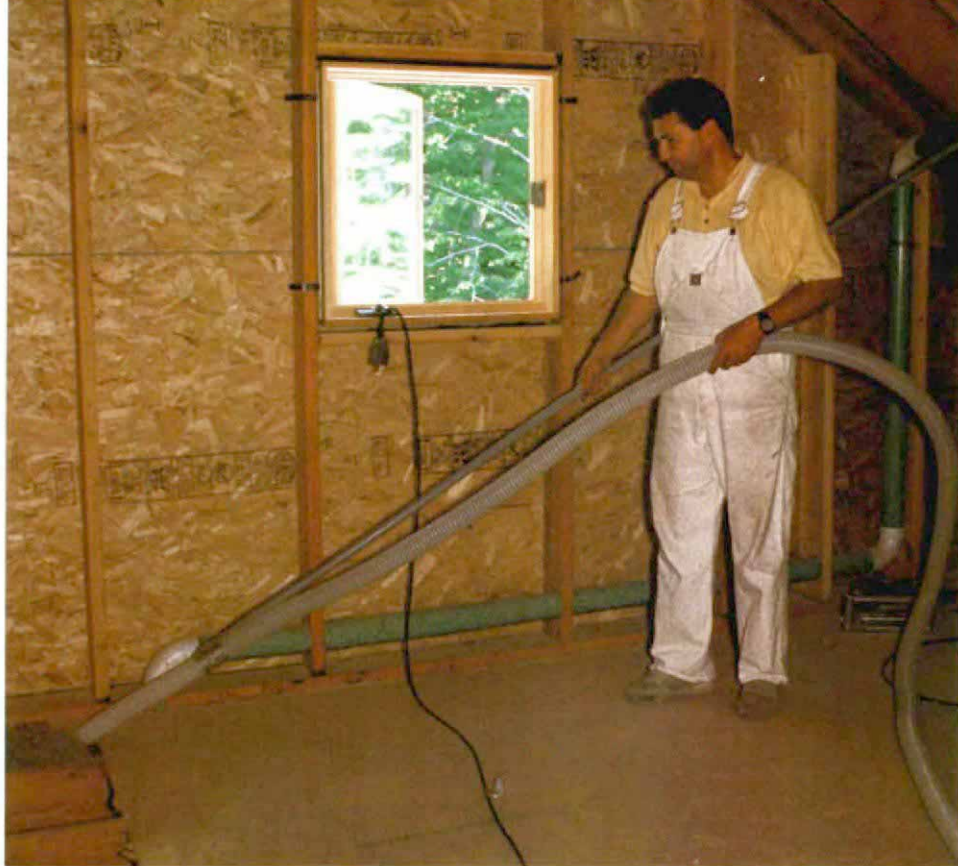
A guide rod supports the hose. Simply 1-in. conduit duct-taped to the hose end, guide rods can be joined together to coax floppy hoses deep into building cavities.
