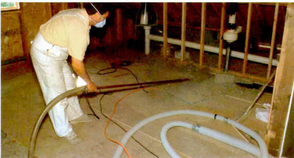
Cellulose can blow into tight spaces. Here, the author has reduced the original 3-in. hose to 1-in. pipe that he's worked into a tight attic bay.
