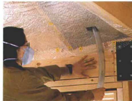
When rigid sheathing isn't practical, membranes can work. They won't hold the density that sheathing can, but membranes seal irregular areas more easily.
