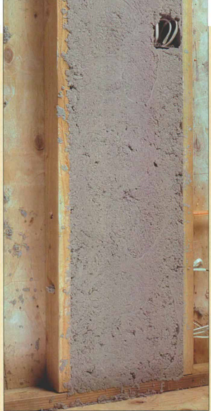
3. Dense-packed to R-3.5 per in., and also air-sealed.
