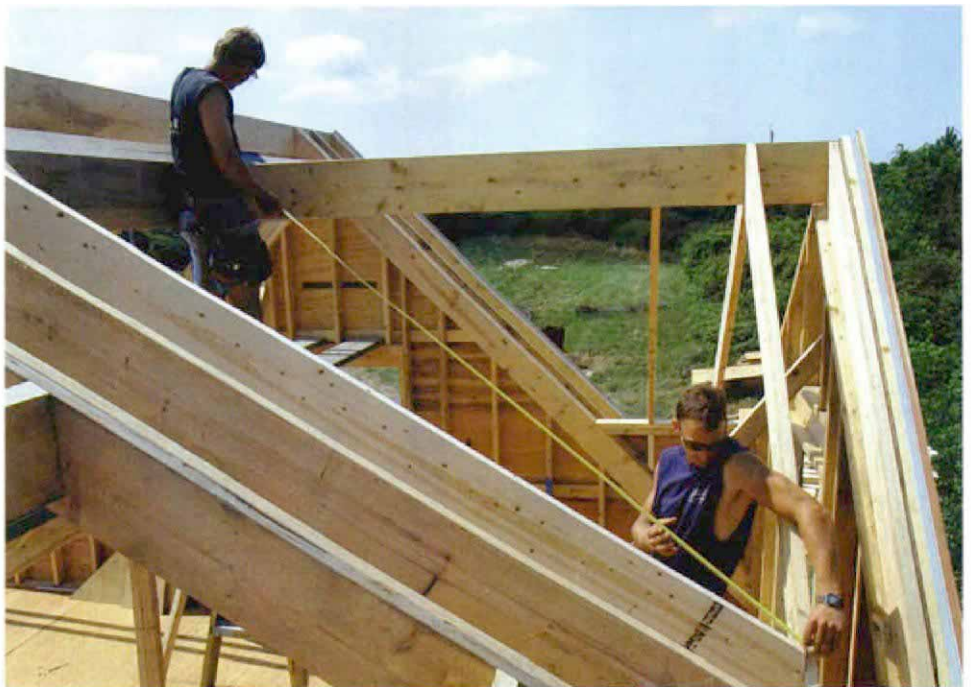
Measuring an irregular valley. The quickest way to figure out the irregular valley is to stretch a line from corner to corner. Here, a measurement is taken along that line.
