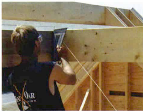
Finding the plumb cut. A rafter square held in the corner against the string determines the angle of the valley plumb cuts.
