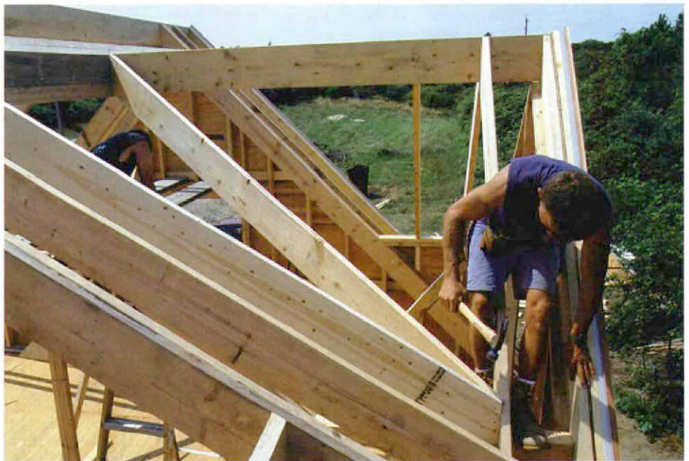
Valley rafter slips into place. After all the angles have been cut into the valley rafters, including a bevel on the bottom edge where the ceiling planes intersect, the valleys are nailed in permanently.
