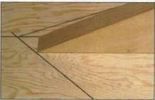
Cutting a bit extra from the seat of a hip or ledger will align it with the roof plane. A plumb line raised where the held-in-place rafter intersects the bay's perimeter (top) shows how much to cut off the rafter (bottom). Unlike beveled rafters, sheathing contacts only the dropped rafters' edge.
