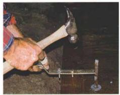
**Anchor-bolt marker.** Lay the plate exactly on the opposite side of its chalkline, center the bolt in the marker, and then whack it with a hammer to mark where to drill the plate. The second bolt is for 2x6 plates.
