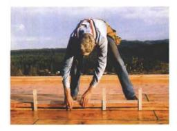
**Layout stick.** With tabs on 16-in. and 24-in. centers, a layout stick locates studs fast. The longer teeth come into play when plates are laid side by side and are marked on their faces rather than edges.
