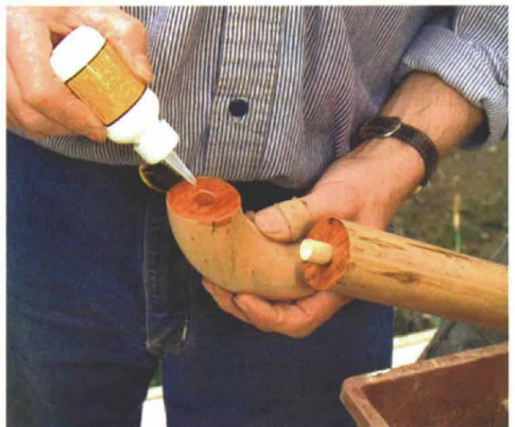
Fitting the end returns. If wall variations make the return stick past the rail (left), that amount is removed. The return is then set in place and indexed to the railing with pencil marks (right) for alignment during assembly. All surfaces including the dowel are coated with glue (below), and the parts are joined together.
