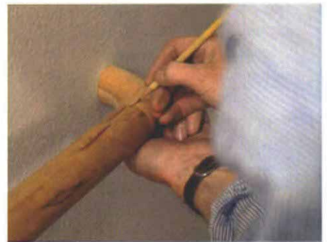
Fitting the end returns. If wall variations make the return stick past the rail (left), that amount is removed. The return is then set in place and indexed to the railing with pencil marks (right) for alignment during assembly. All surfaces including the dowel are coated with glue (below), and the parts are joined together.
