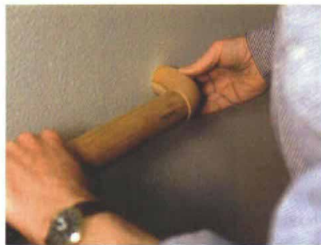
Fitting the end returns. If wall variations make the return stick past the rail (left), that amount is removed. The return is then set in place and indexed to the railing with pencil marks (right) for alignment during assembly. All surfaces including the dowel are coated with glue (below), and the parts are joined together.
