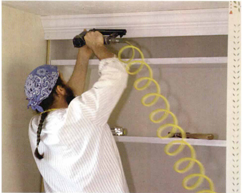
Crown hides ceiling discrepancies. The first trim to be installed is the crown backer and molding, which is adjusted to disguise a ceiling that is out of level.
