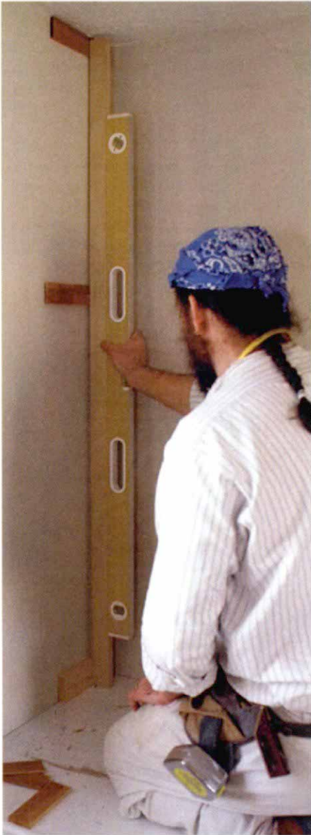
Shims set before the sides go in. Using a straightedge and a level, the author tacks shims to the wall to create a plumb line before the sides are fit.
