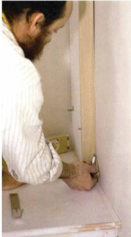
Compass scribes handle larger differences. For big irregularities such as the ones here, inexpensive but invaluable compass-style dividers transfer the wall's contour to the piece being fitted.
