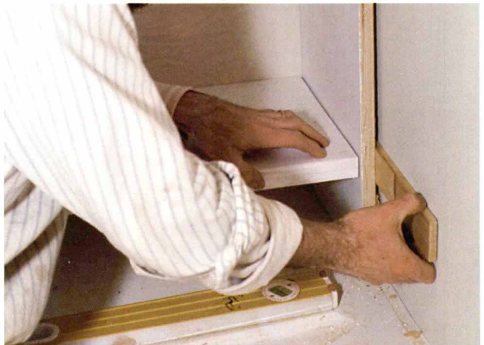
Scribing with a pencil. To scribe variations of less than \frac{1}{8} in., the author lets a pencil ride on the wall, its point recording the scribe line.
