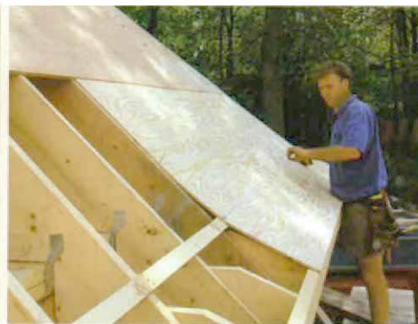
Snapped line guides the fasteners.
