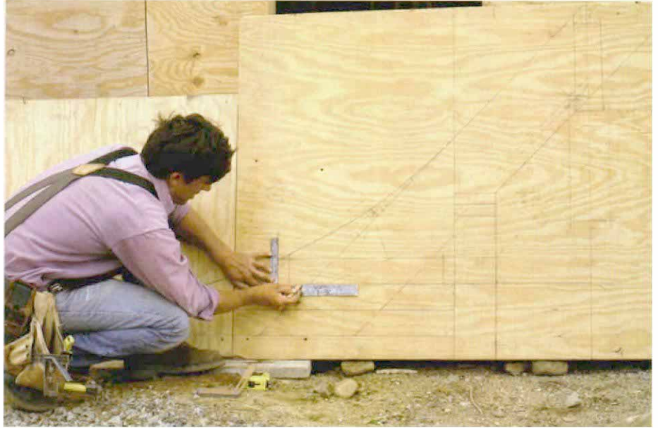
Full-scale drawing determines framing.
