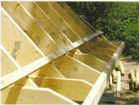
Continuous cleat anchors the curve.
