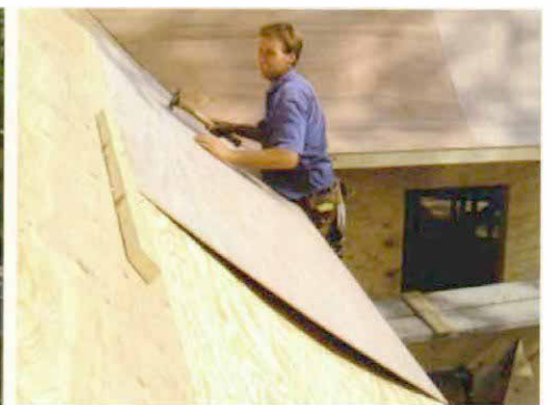
Two layers of plywood bend more easily.
