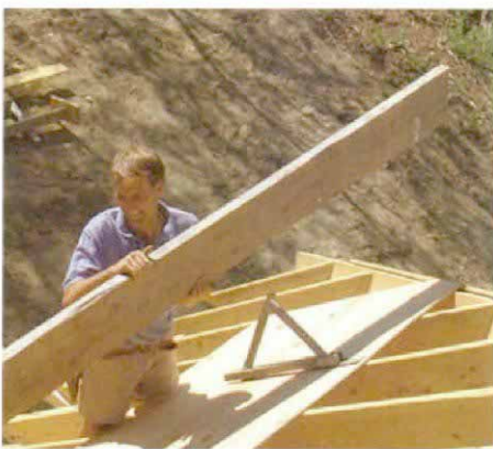
Staging goes on before the courses go up. After the first course of sheathing is nailed off, roof brackets are nailed in and planks are set before the next course is started. Staging provides a safe place to stand as well as a place to rest the sheets for the next course.
