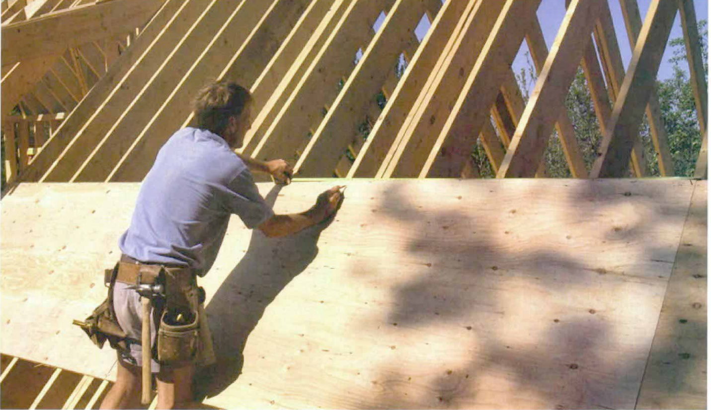
The sheathing straightens the rafters. Before nailing off the sheathing, a tape is hooked to the rafter on one end, and the rafter layout is marked along one edge. The rafters are then moved to the mark and nailed in place.
