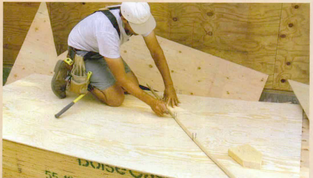
Double nails hold the batten to the curve of the hip.
