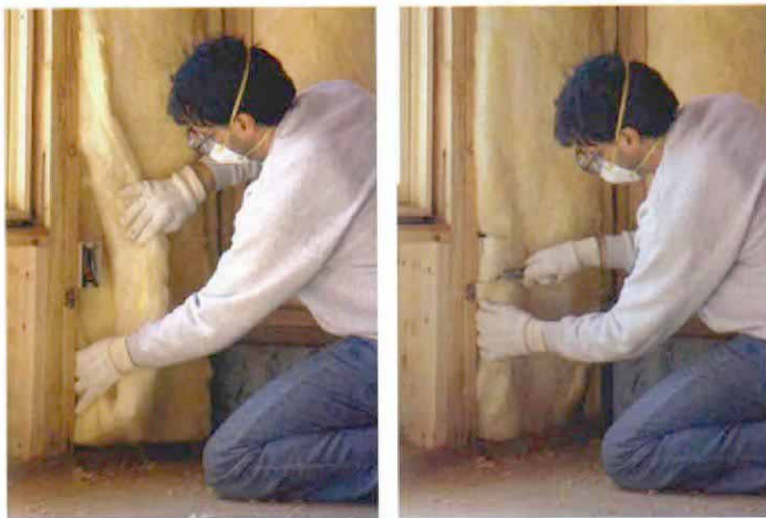
Insulate behind electrical boxes. To get fiberglass behind an electrical box, split the batt vertically (photo left), hold the remainder over the box and cut around the outside of the box (photo right).
