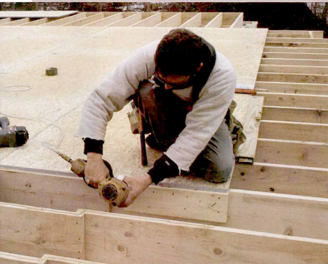
Added support at the overlap. The joist layout changes wherever the joists overlap at an interior bearing wall or a carrying beam leaving part of the edge of the sheathing unsupported. A 2x block is nailed in to hold the unsupported edge (photo above), and the layout is clearly marked for accurate nailing (photo right).
