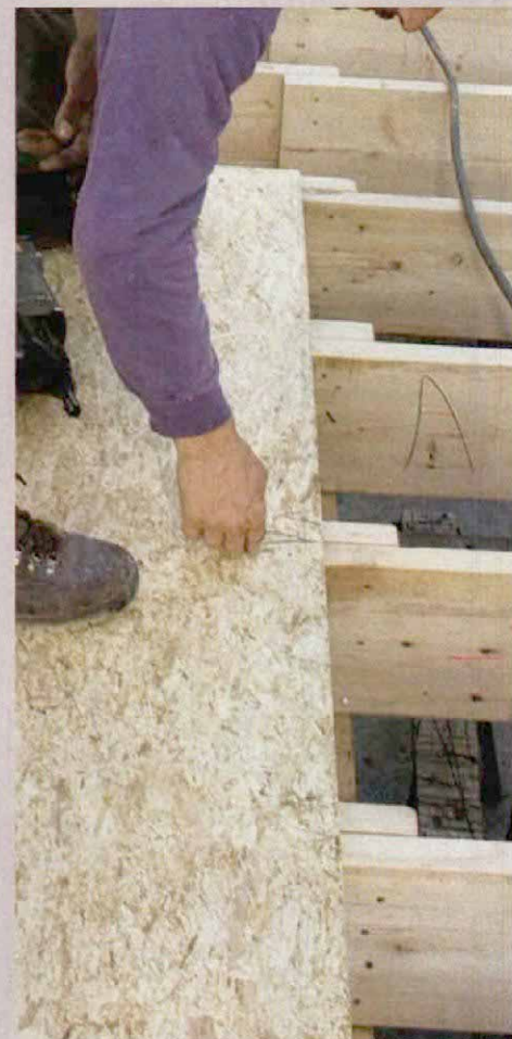
Added support at the overlap. The joist layout changes wherever the joists overlap at an interior bearing wall or a carrying beam leaving part of the edge of the sheathing unsupported. A 2x block is nailed in to hold the unsupported edge (photo above), and the layout is clearly marked for accurate nailing (photo right).
