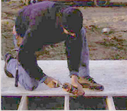
Start spreading the glues. A generous bead of construction adhesive is spread on each joist and on the plywood edge.
