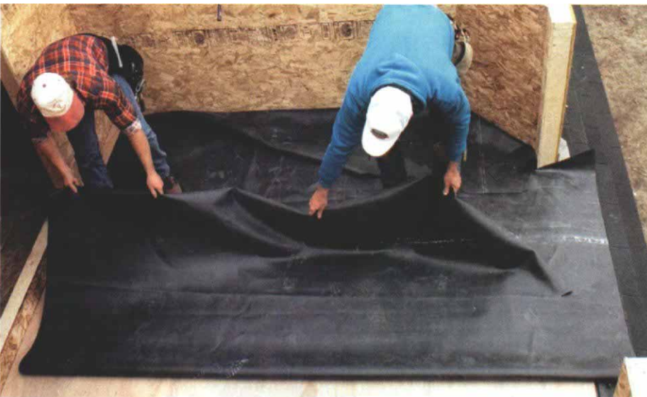
Unrolling the membrane for a dry fit. After the substrate has been prepared properly, the sheet of EPDM is laid out in the area to be covered for a dry fit.
