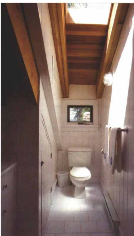
K. Toilet strategically placed between rafters.
