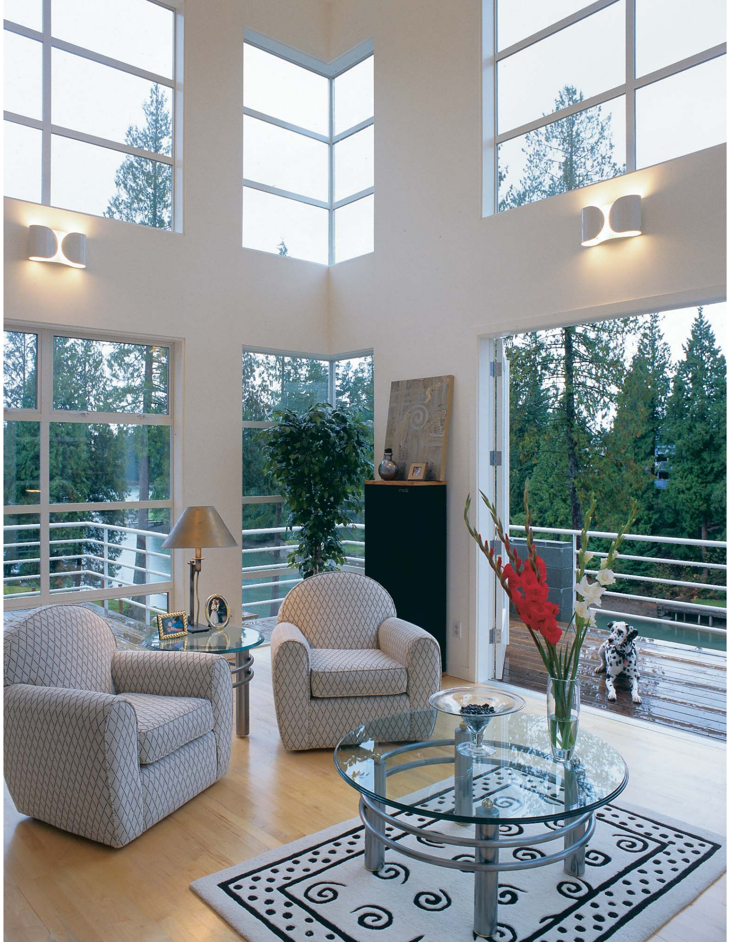
There's more keeping these walls stiff than meets the eye. Buried within the shear-paneled framing of this two-level living room is a steel wind beam that separates the top tier of windows from the bottom.
