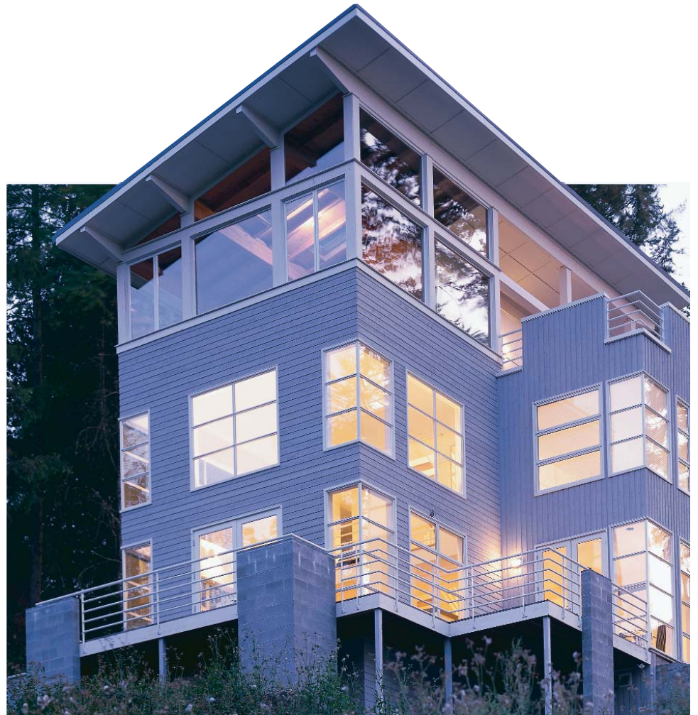
More than one-third glass. With its roof at a dapper tilt and with 35% of the walls covered with glass, this lakeside house near Seattle needed more than conventional framing to keep it from shifting in high winds.
