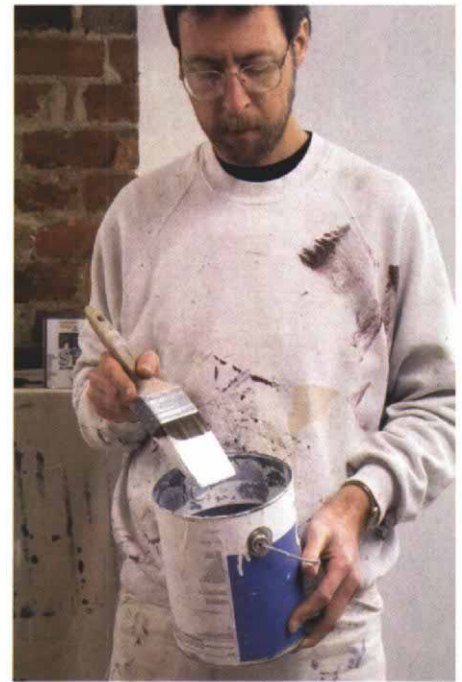
Keep your other hand out of the way. To hold the cut bucket, hook your thumb in the handle with your fingers locked under the bucket. This grasp lets you load the paintbrush without interference.
