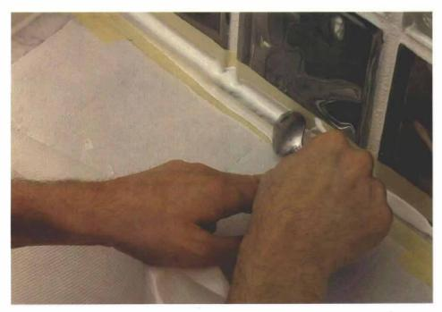
A spoon can get into a tight spot. A spoon that has a fairly tight radius on the tip can create just about any type of cross section, even a wide joint such as the one around this glass-block window. Sometimes it's necessary to mask around the bead with tape.
