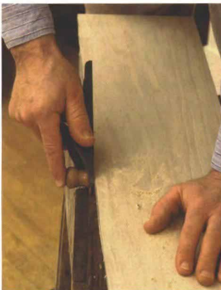
A block plane fine-tunes the scribe. Having back-cut the baseboard with the jigsaw, planing (with the plane held square to the face) is easier because there's less stock to remove.
