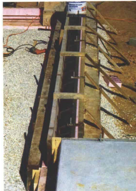
Insulation extends beyond the stemwalls. Garage stemwalls are formed directly on top of the foam-board insulation. The insulation continuing beyond the stemwall perimeter traps heat from the earth to keep frost at bay.
