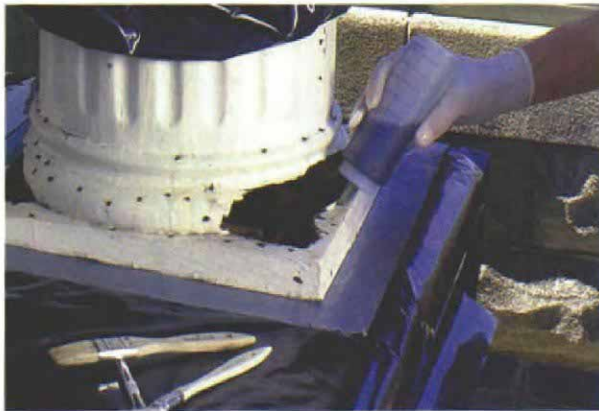
Brushed-on epoxy consolidates exposed wood. In addition to being injected, consolidant is brushed onto exposed wood until it no longer soaks into soft wood.
