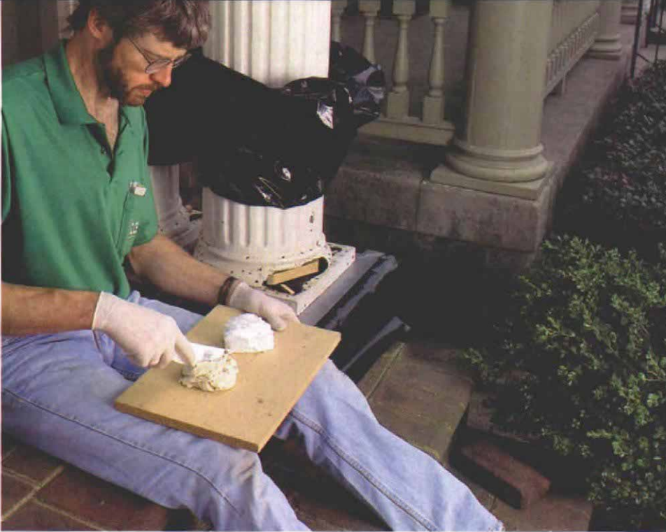
Two-part fillers are mixed on a board. After measuring the right amount of resin and hardener paste, the two are kneaded together on a scrap of plywood.
