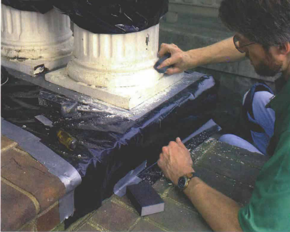
Woodworking tools also handle epoxy. Cured epoxy can be worked like wood. A chisel and a Surform plane rough out the shape, and sandpaper does the smoothing.
