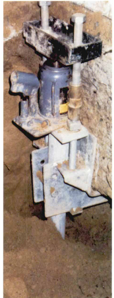
Brackets strong enough to hold up a house. Brackets that tie helical piers to the foundation are designed to accept a heavy-duty hydraulic jack (photo above). With several piers sharing the load, a section of a house can be supported or lifted (photo left). As the foundation is raised, nuts on the bracket are tightened, locking the bracket in place.
