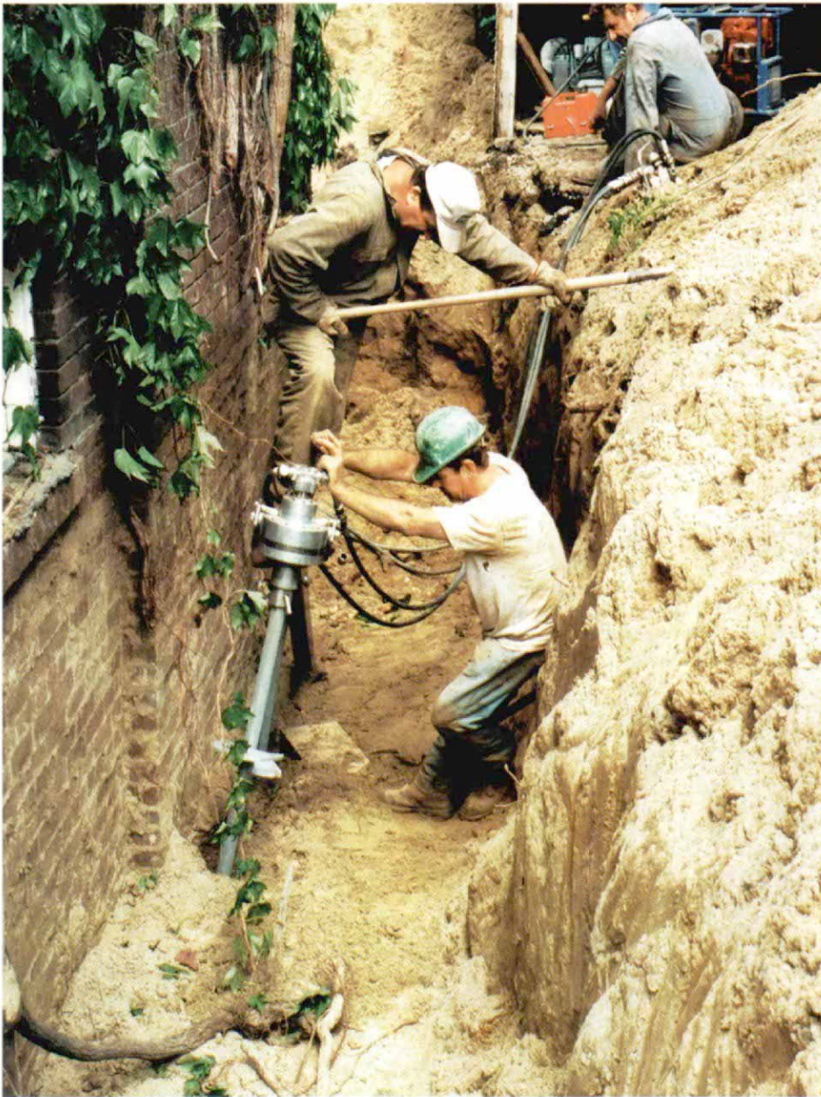
A big wrench drives the piers. Two installers from W. C. Pietz Ltd. of Toronto drive a helical pier next to a foundation wall using a hydraulic motor called a power, or digger, head. The installer above is standing on a support arm, similar to a huge ratchet-wrench handle, to help to keep the power head from turning.
