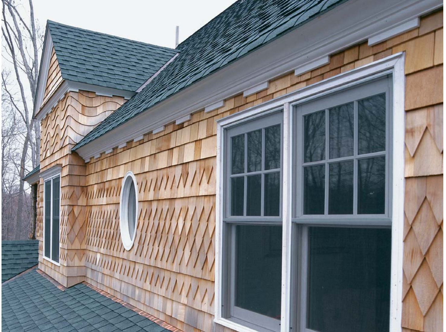
A traditional profile that performs a modern function. This crown-and-dentil eave provides nearly as much ventilation to the rafter bays as a continuous aluminum soffit vent.
