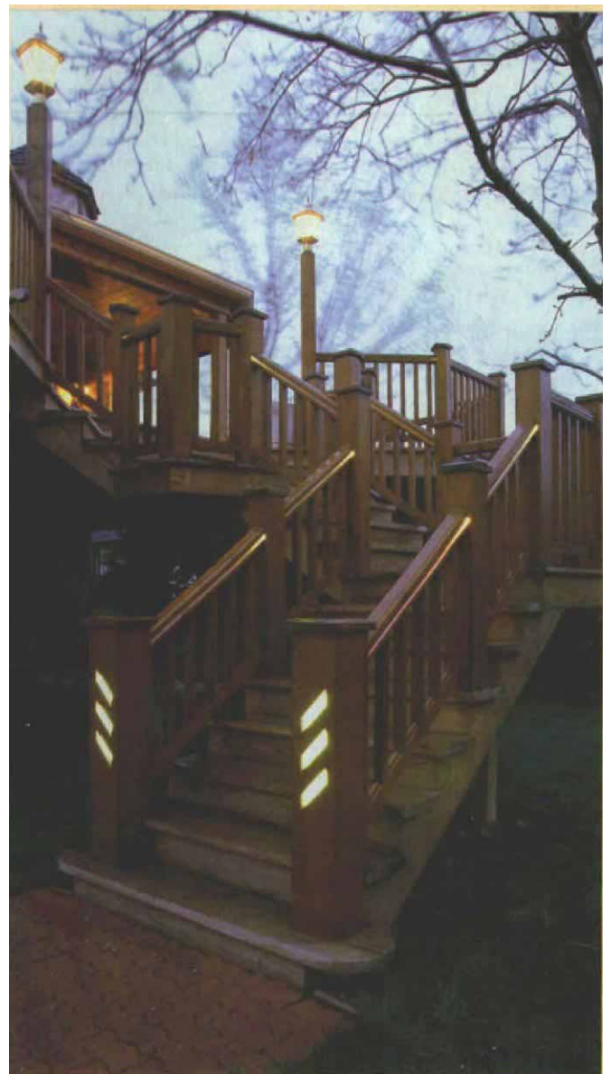
Acrylic rods help to light the way. Inset into the handrails, solid acrylic rods reflect light from fluorescent fixtures concealed in the newel posts.
