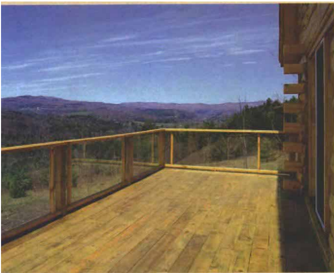
A glass railing doesn't obscure the view. Salvaged tempered-glass panels from failed thermopane sliders make a strong and unobtrusive deck railing.
