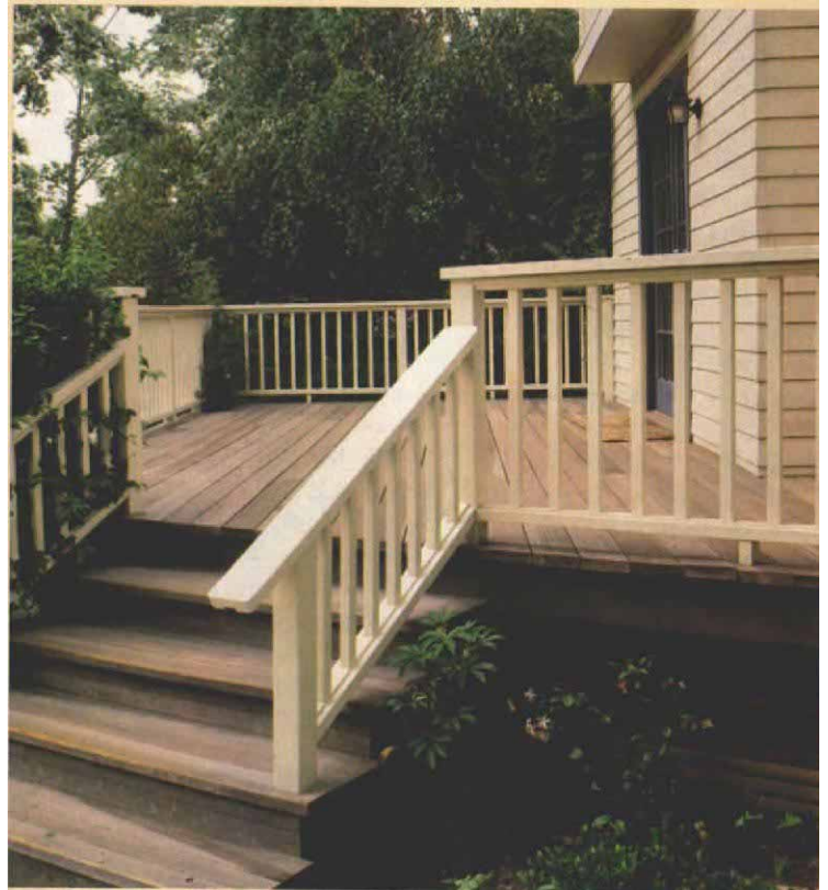
Slip tenons reinforce this redwood railing. The bottom rail on this redwood railing drops onto slip tenons mortised into the posts. The balusters are premounted onto ¼-in. by 1½-in. battens to make a balustrade that is then attached to the top and bottom rails.
