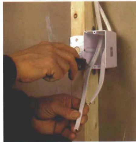
A utility knife slits the sheathing. Leaving about ¼ in. of sheathing coming into the box, slit the sheathing carefully along the flat side of the cable to avoid damaging the wires inside. Then peel the sheathing back and slice it off carefully inside the box.
