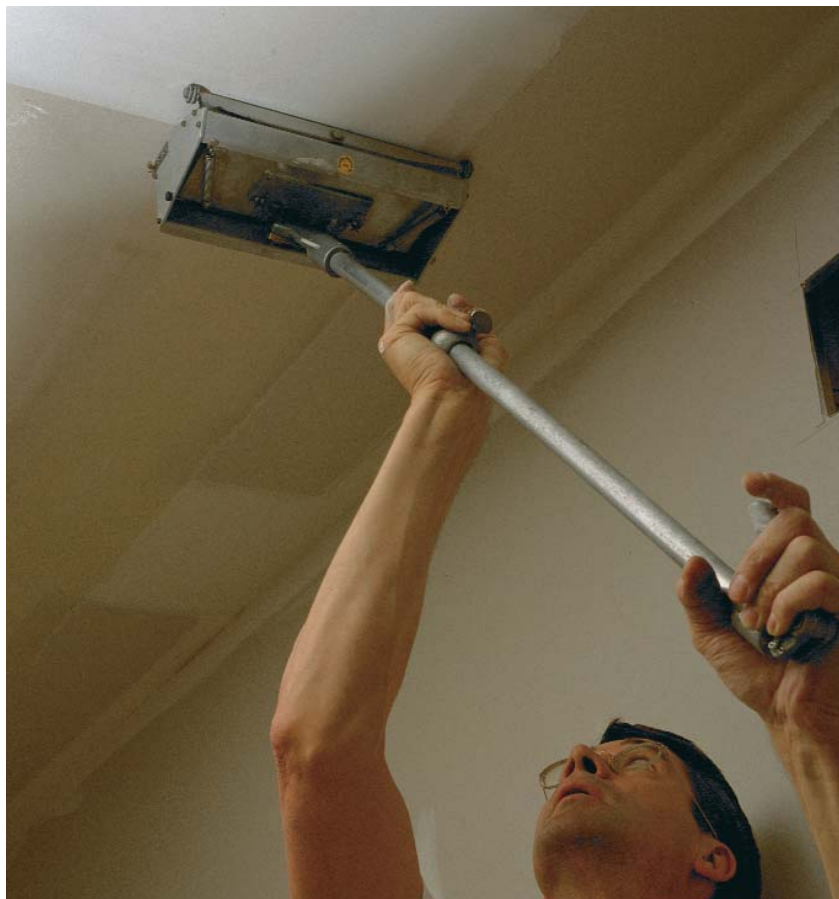
Adjust the blade to control crowning. A dial on this flat finisher sets the curve of the blade, which determines how big the crown will be on the top coat of joint compound.
