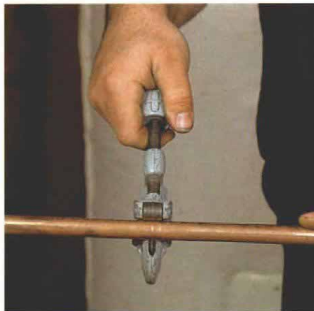
Tubing cutter must be square to pipe. Align the cutter by tightening the handle and making a couple of revolutions. If the cutter is staying in its groove, continue the cut, tightening the handle every couple of revolutions.
