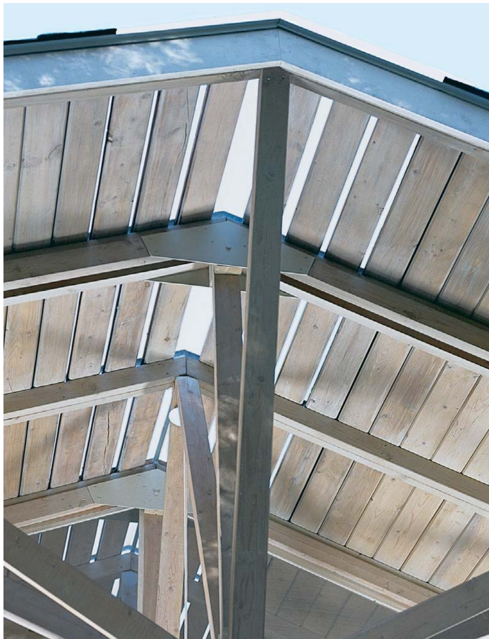
He didn't run out of roofing boards. Because the roof has such deep overhangs, a ridge skylight was needed to brighten the porch. This unconventional skylight is a series of progressively wider gaps between roofing boards, all covered with a Lexan ridge cap. The trusses and 2x6 roof boards are finished with semitransparent stain similar to the gray of the floor and the stonework.
