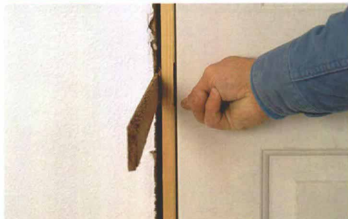
10. Equalize the strike-jamb reveal. Use shims placed next to the door latch to adjust the strike jamb in or out until the gap is consistent from top to bottom.
