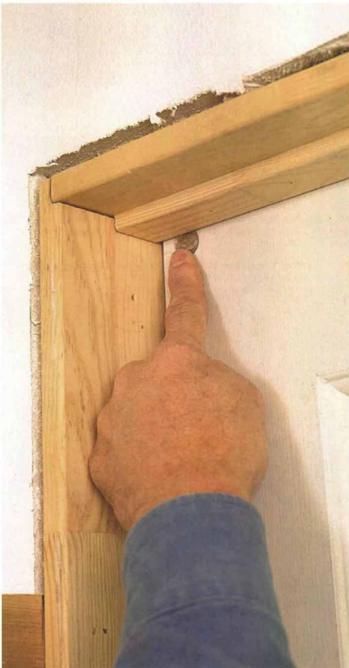
12. Don't forget the stop gap. Use a dime between the closed door and the doorstop to gauge a consistent gap between the door and the stop. The gap allows for paint buildup.
