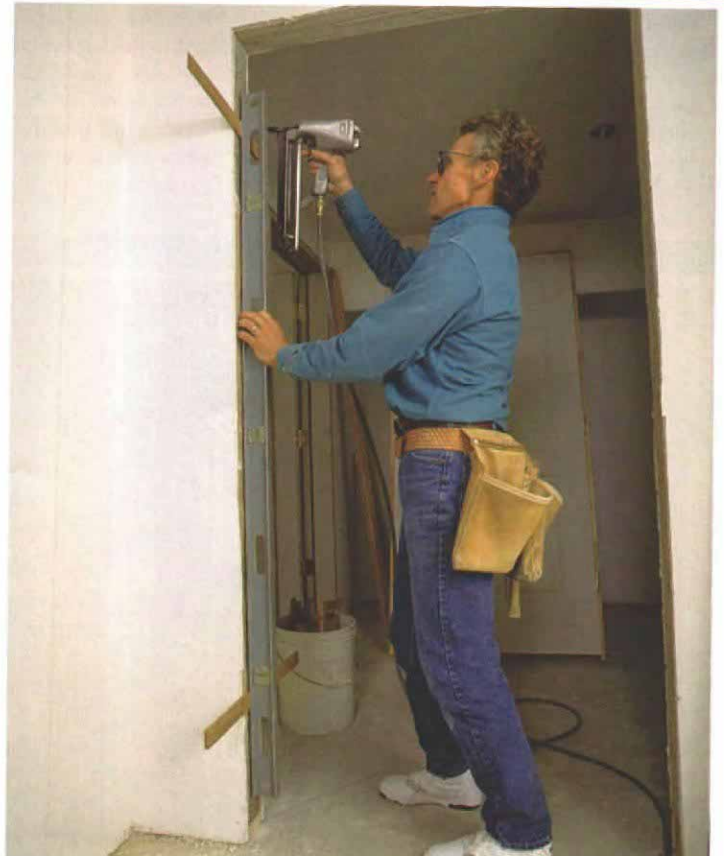
5. Affix the shims. Shims behind the top and bottom hinges make backing for the jamb. A single shim at the top compensates for twist.
