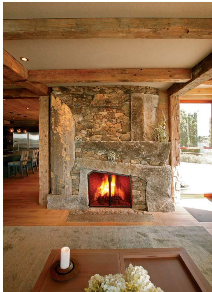
Master mason. Lew French is the craftsman behind all of the home's stonework. Using granite from old New England foundations and recycled fieldstone, Lew carefully selects and places each stone, rarely cutting or altering that rock. (For more on Lew and his work, see p. 106.)
