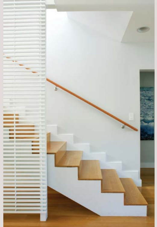
The 7/11 stair. The new stair is based on a rise of 7 in. and a run of 11 in., similar to that found at the entrance of a library. This makes for a deeper but more comfortable set of stairs.
