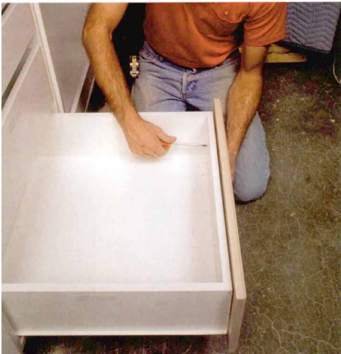
Fitting a drawer front. Drawer fronts in a European-style kitchen must be installed accurately. Two threaded, adjustable inserts are let into 20-mm holes in the back of a drawer front (above), which is then attached to the box with machine screws run into the inserts (below).
