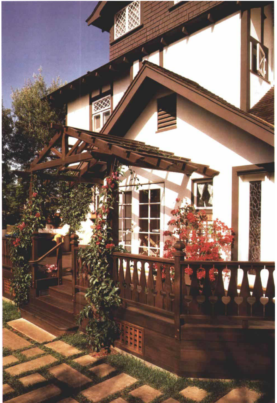
Deck complements house. A timber-frame pergola, closely spaced balusters and an enclosed crawlspace—all made of redwood that’s been stained dark—make this deck appear as if it were always part of the Tudor-style house.
