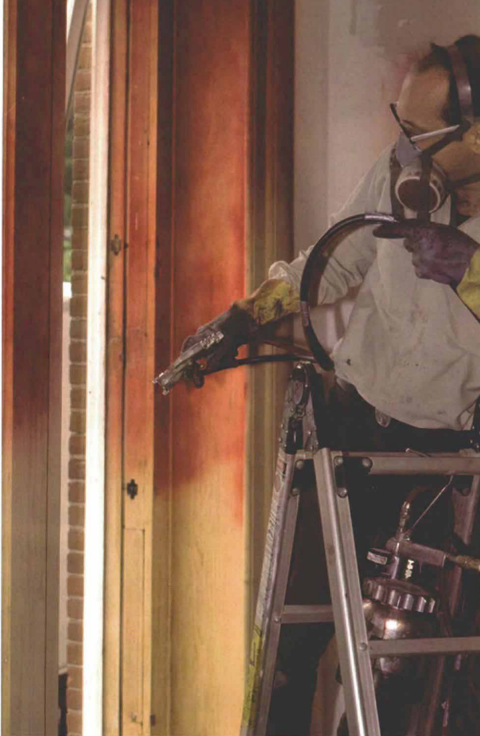
Base coat applied. The first layer of color, a red NGR dye, is an alcohol-based dye that won't raise the grain of the wood. A dye concentrate is thinned with methanol and sprayed on with a standard air gun to match a color sample that was made up in advance.
