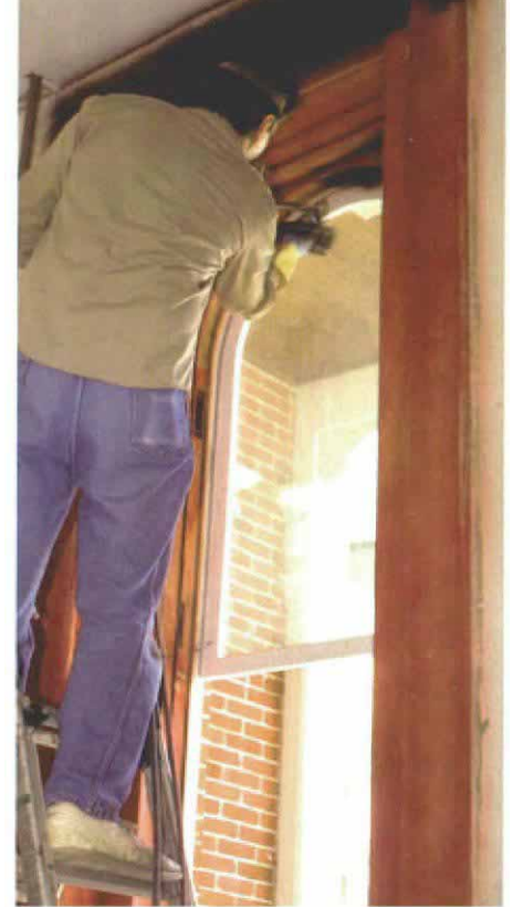
Adding a second color gives depth. After the base color has dried and a wash coat applied, a solvent-based stain is sprayed on. This second color is allowed to penetrate the wood and then is wiped off with a lint-free cloth or a dry China bristle brush.
