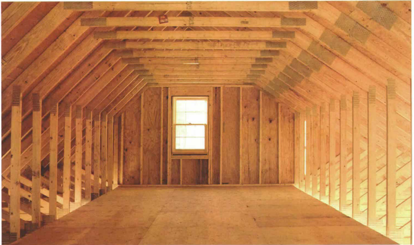
Attic storage with a truss. Not all trusses eliminate attic storage or attic-level living spaces. Attic trusses carry extra loads on the bottom chord and provide a room-size cavity between webs.
