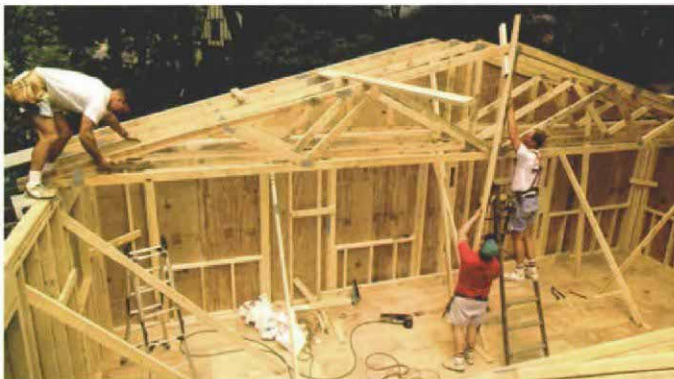
For small trusses, poles will do. First-floor trusses with relatively short spans can be poled up. Supported by two outside walls (top), trusses are rolled upright with a Y-shaped pole (middle). When the truss is plumb, it must be braced to other trusses and toenailed in place. In this installation, the use of two poles would have been better.
