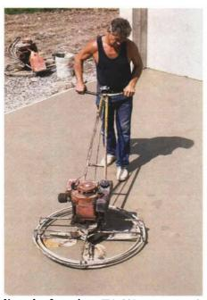
Note the footprints. This 36-in. power trowel has four rotating combination blades that float and finish a concrete slab. The operator walks backward and erases his footprints with the machine.
