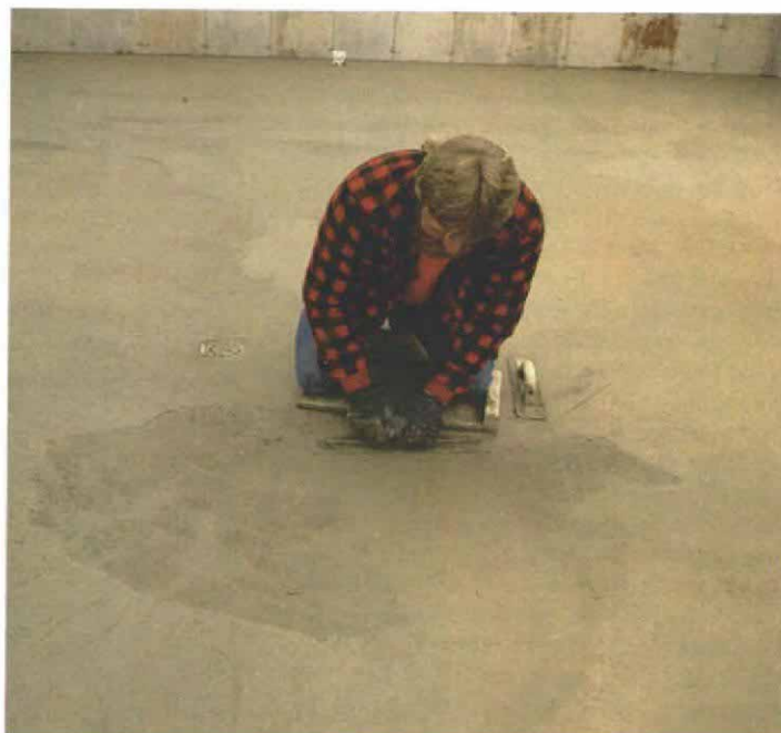
Two hands! Two hands! As the concrete sets up, working it with a steel trowel may require the strength of two hands. The back of the trowel is angled up as you push it away (left), and the front of the trowel is angled up as you pull it toward you (right).
