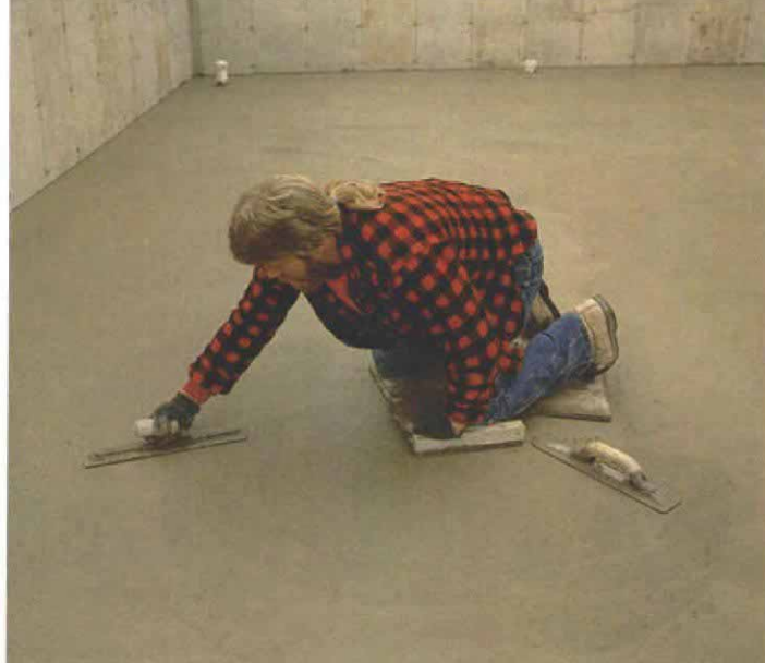
Start with a mag; finish with steel. After bull floating, use a magnesium float (left) to smooth out bumps and fill in low spots. The resulting finish will be coarse. Later, use a steel trowel (right) to get a smooth, dense finish that won't crumble when it's swept.
