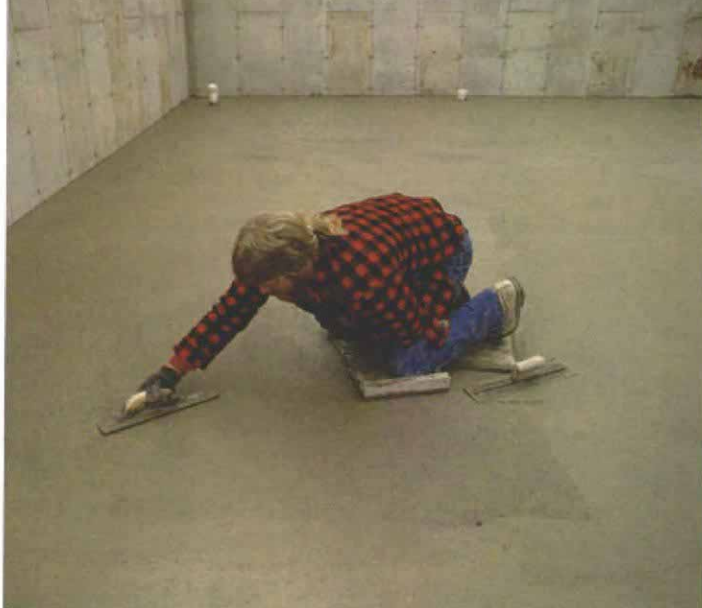
Start with a mag; finish with steel. After bull floating, use a magnesium float (left) to smooth out bumps and fill in low spots. The resulting finish will be coarse. Later, use a steel trowel (right) to get a smooth, dense finish that won't crumble when it's swept.
