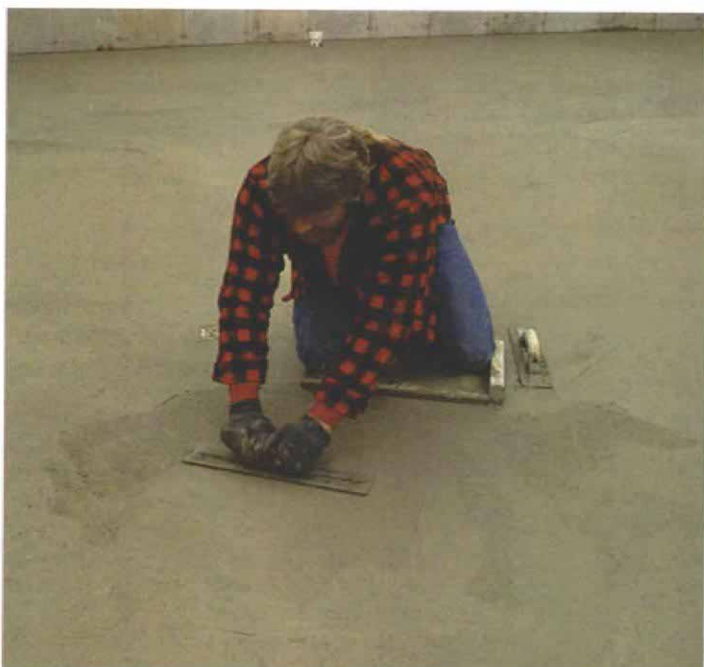
Two hands! Two hands! As the concrete sets up, working it with a steel trowel may require the strength of two hands. The back of the trowel is angled up as you push it away (left), and the front of the trowel is angled up as you pull it toward you (right).
