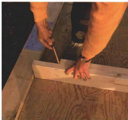
Scribing the jacks. By holding a stud alongside the king stud and against the underside of the header, the jacks can be scribed without measuring. Visible on the bottom plate, half hidden by the carpenter's hand, is a galvanized plate nailed over joints in the plate.
