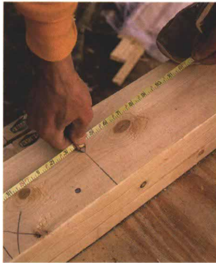
Layout trick. A flexible wind-up tape is used for layout. Hold a pencil against the tape and swing it across the plate to make marks. The farther the tape is away from the end of the plate, the straighter the lines will be.
