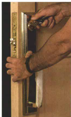
14. Use a key to tighten the dead-bolt cylinder.
