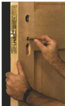
12. Threading in the knob spindle from exterior.
