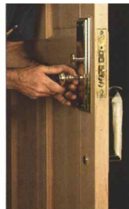
16. Threading the knob onto the spindle.
