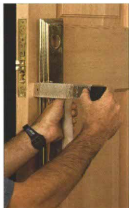
13. Measuring the thumb-lever shaft.
