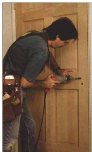
10. Drilling the interior layout.
