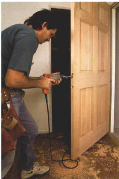
2. Drilling a series of overlapping holes.
