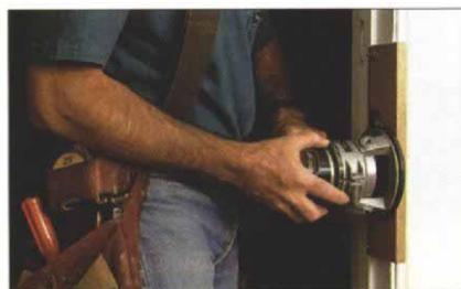
17. Making a shallow strike-plate mortise.
