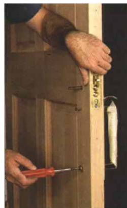
15. A mounting screw secures bottom of handle.
