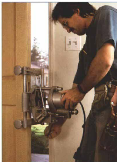
5. Using the lock mortiser.
