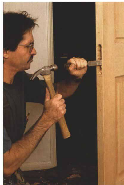
3. Shaving the mortise clean.
