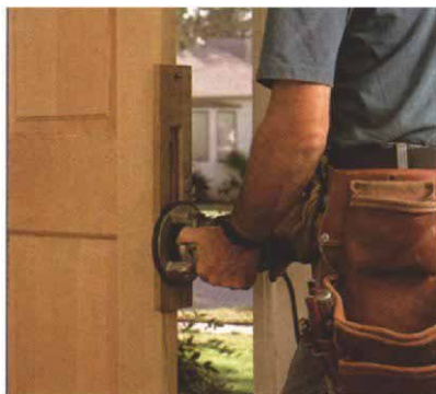
6. Routing for the latch plate.
