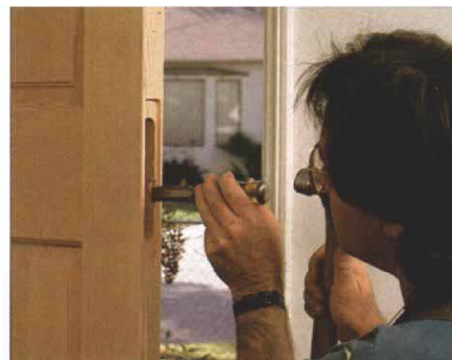
7. Notching for the latch hinges.
