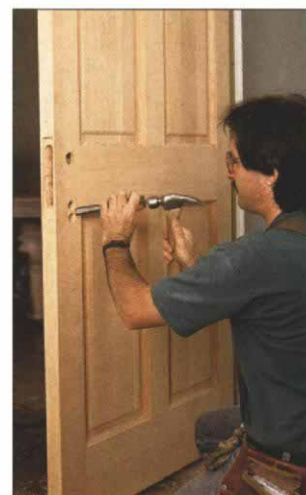
11. Chiseling keyhole mortise.
