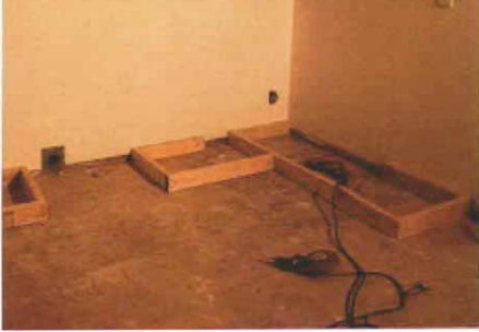
First the frame. The author assembled the base cabinets atop a frame of 2x4s toenailed to the wall and the subfloor.
