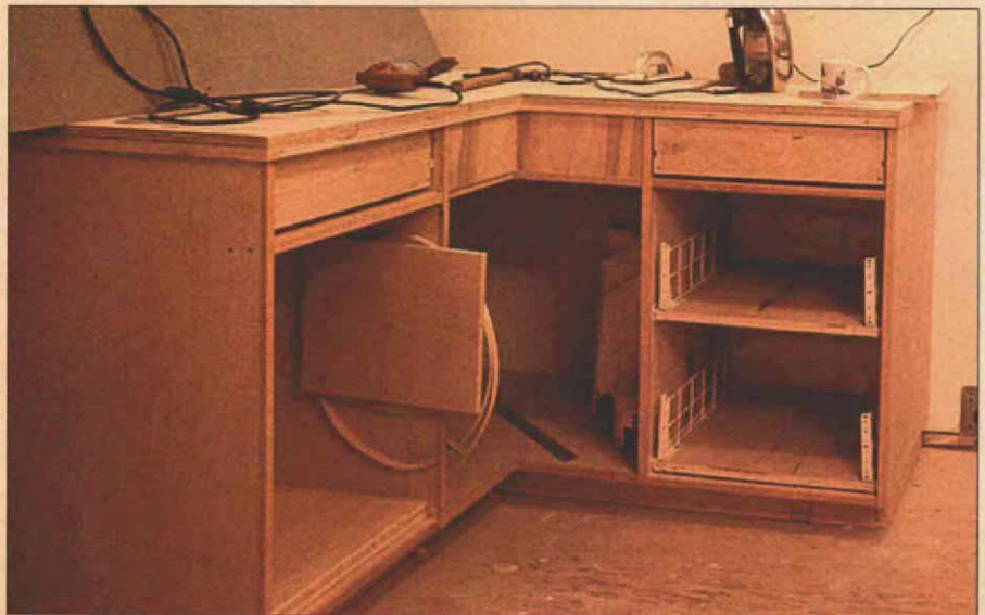
Under the doors and the drawer fronts. Shallow drawer boxes ride on wood runners affixed to the cabinet partitions and end panels. The lower drawers on the sink-side base cabinets are commercial bins that use roller hardware.
