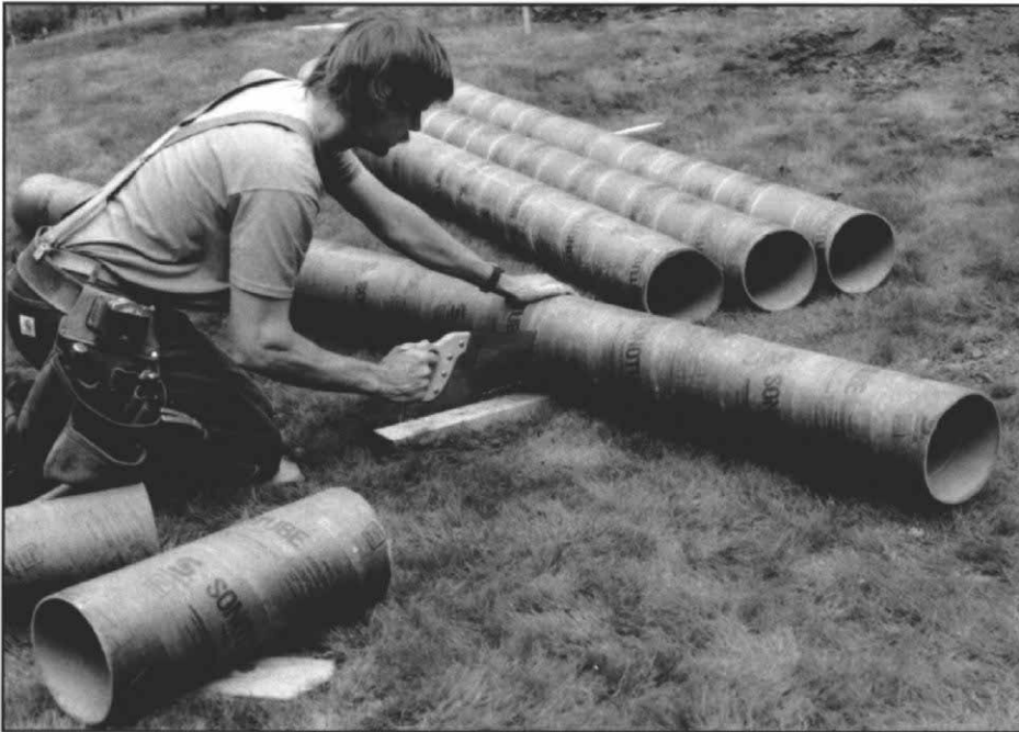
Form cutting made easy. One advantage of using round fiberboard forms is that they are easily cut to length. Just use a handsaw, but try to make the cut square.
