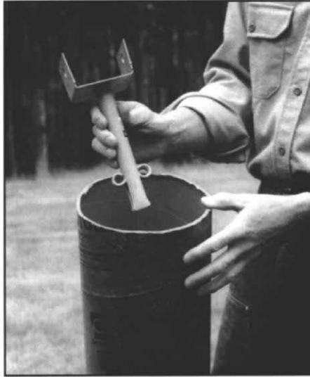
Post connectors. There are several types of metal connectors that can be used to attach wooden posts to concrete piers. This one is placed in wet concrete.
