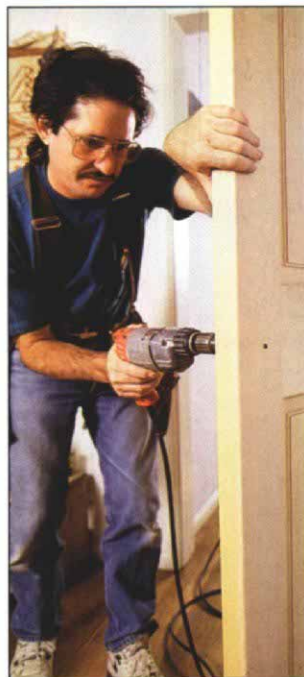
3. Stop drilling when tip emerges from opposite side.
