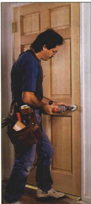
2. Start facebore, aligning hole saw with center of lock rail.
