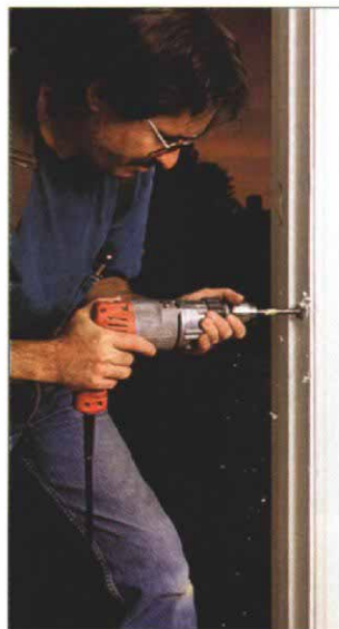
15. Drill the latch hole in the middle of the penciled outline.
