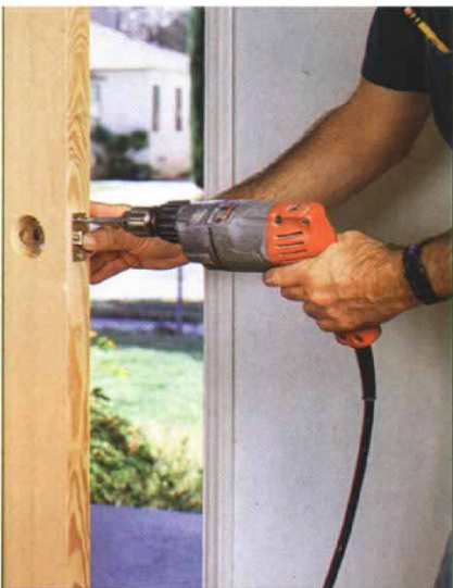
21. Install the latch before the knobs.
