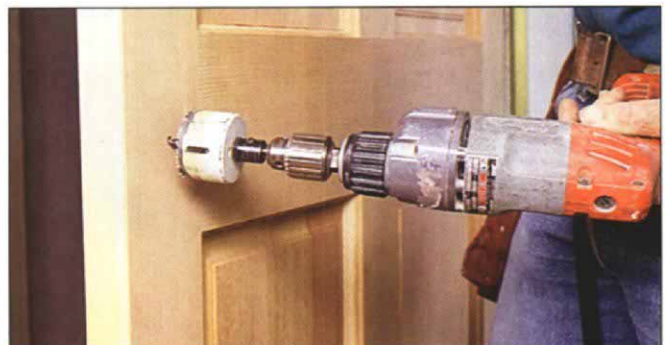
4. Finish facebore from other side; use hole to guide mandrel bit.
