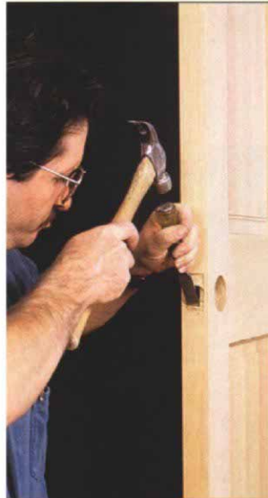
12, 13. Chisel out the scored mortise from center to bottom and then finish it by chiseling up from the center.
