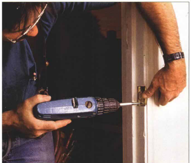
16. To prevent screws from splitting the wood, drill pilot holes.
