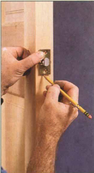
10. Insert the latch and trace the latch-plate outline.
