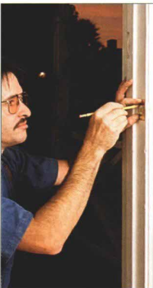
14. Trace the strike plate and the latch opening.
