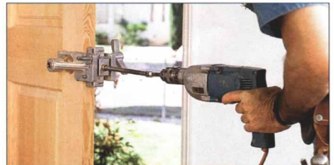
9. A boring jig ensures straight, worry-free edgeboring.
