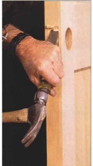
12, 13. Chisel out the scored mortise from center to bottom and then finish it by chiseling up from the center.
