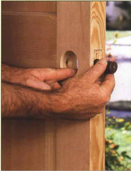
19. Insert the center marker, point out.
