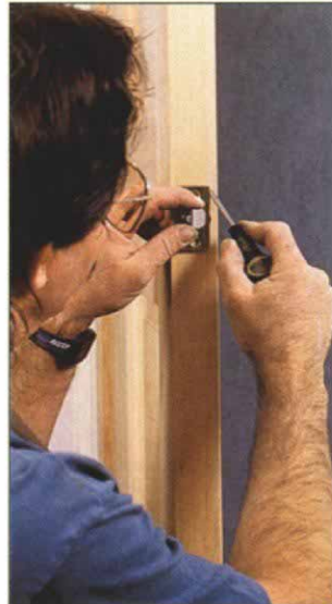
11. Use an awl to score the two edges with the grain.
