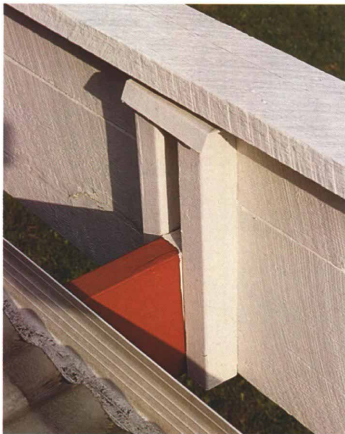
Behind the fascia. Vertical cleats nailed to the joist support the fascia. Flashing and an angled 1x6 protect the fascia boards from runoff.
