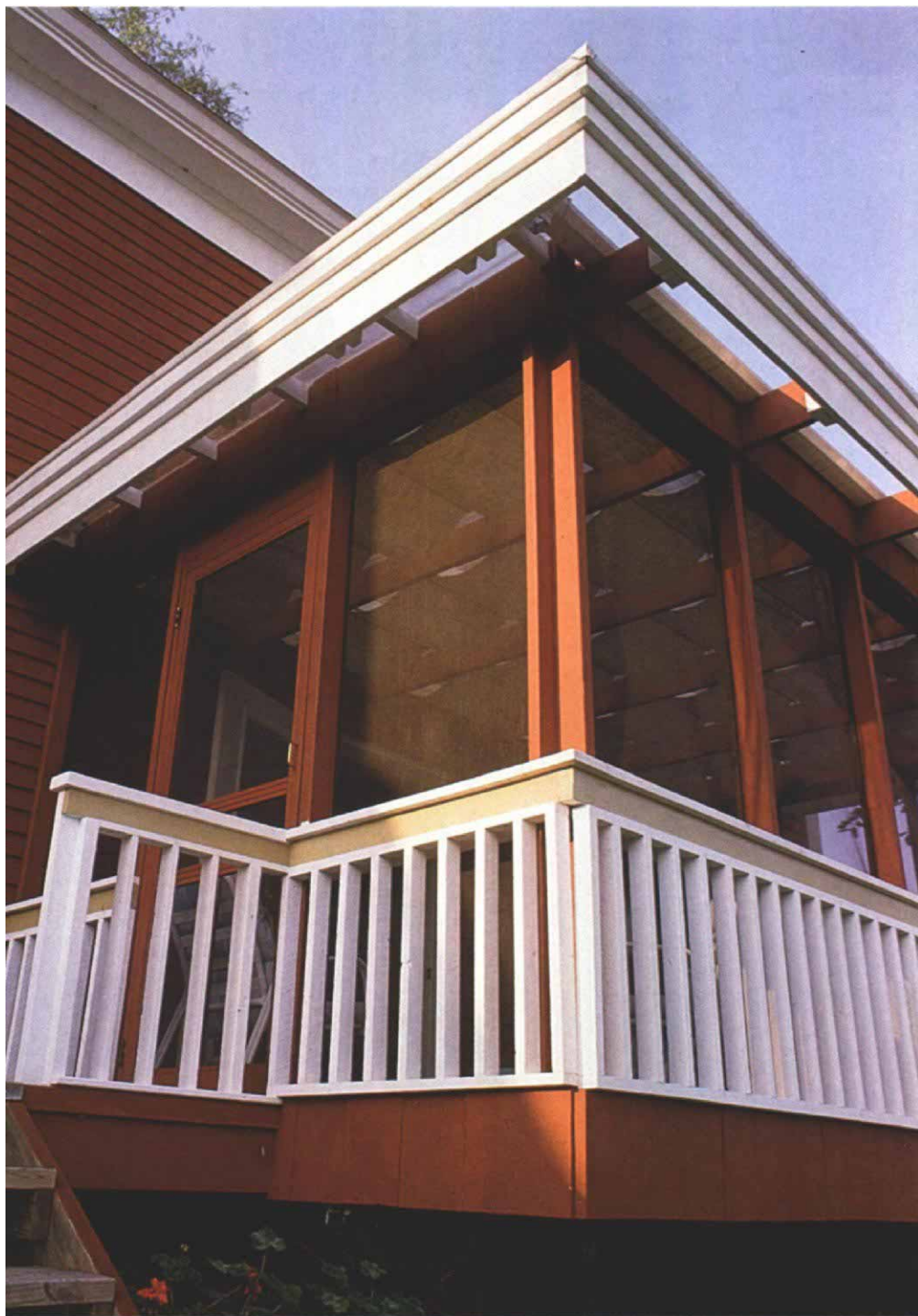
Roof structure. A three-tiered 15-in. fascia conceals a very shallow-pitched shed roof constructed of pressure-treated framing and corrugated, fiber-reinforced plastic (FRP) panels.
