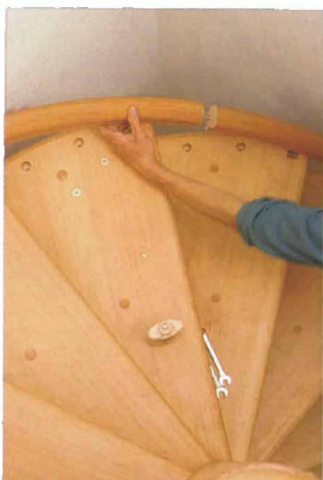
Handrail joint. Handrail sections are joined with a rail bolt. A hole in the underside of the upper rail allows access to tighten a nut onto the bolt's machine-threaded end.
