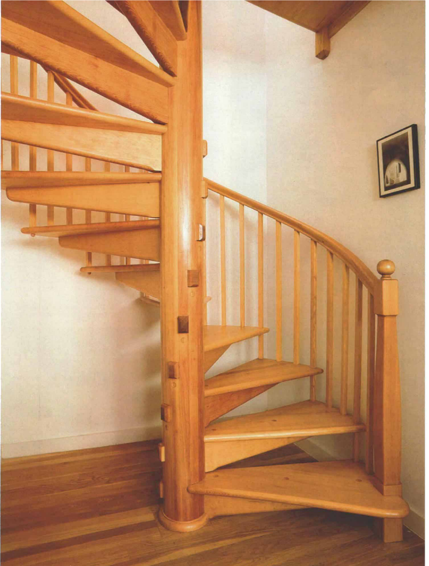
Cantilevered treads. The author's spiral staircase rises on treads mounted atop ribs that extend through a hollow column. The treads wind their way from an enlarged first tread to a second-level landing that is borne primarily by ledgers affixed to the wall.
