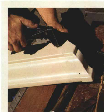
A pop-riveter is an essential tool for miter strips and gutter sections.
