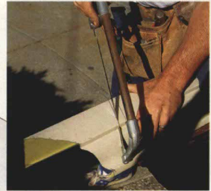
Ogee gutter. Use a hacksaw to cut down the face of an aluminum ogee gutter. Begin at the corner between the bottom and the face, with the saw held at 45°. Finish the cut down the back with tin snips.
