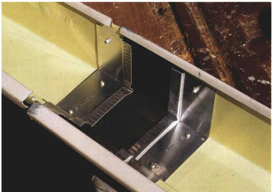
An expansion joint should be installed between sections of gutter more than 40 ft. long, or between fixed corners. Note how the hems have been trimmed off the piece on the left.
