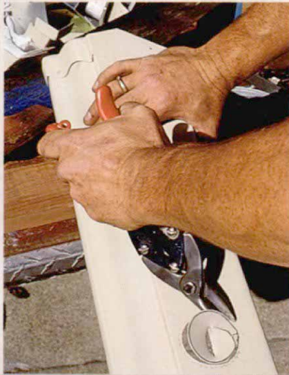
After making an entry slit with a chisel, Williams uses a pair of aviation snips to make a cutout for a downspout outlet.
