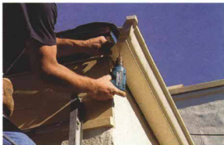
The face of an ogee gutter has an S-curve and a couple of reveals to cast shadow lines. Here the author drills a hole through an outside miter strip prior to pop-riveting the miter strip to the gutter section.
