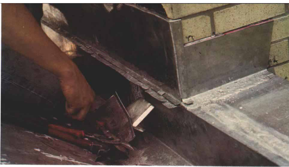
Chimney flashing is held fast in a reglet cut into mortar joints and clipped to the gutter liner at the bottom (photo above).
